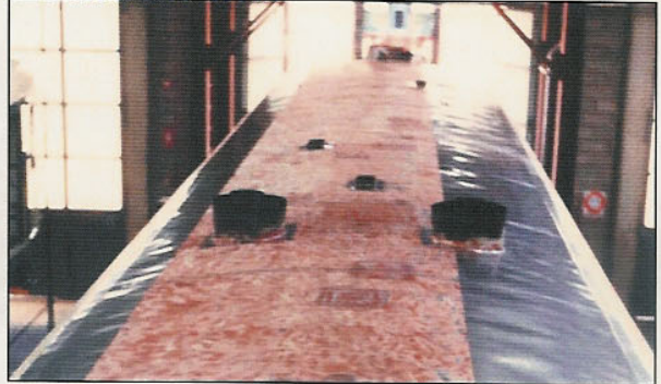
Application of zinc tape on Railway Carriage.
