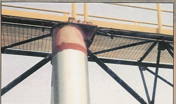
Application of zinc tape on a Bridge Support.
