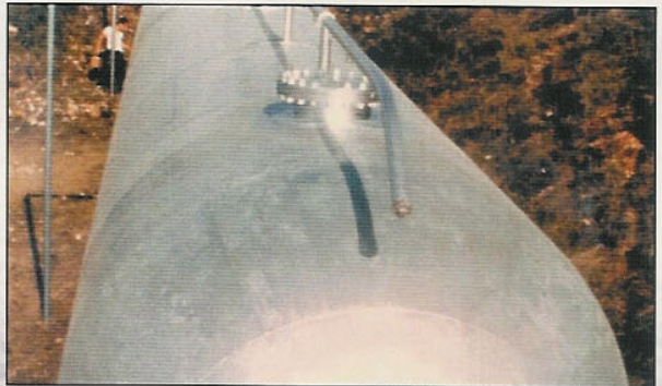
Application of zinc tape on Fuel Tanks.
