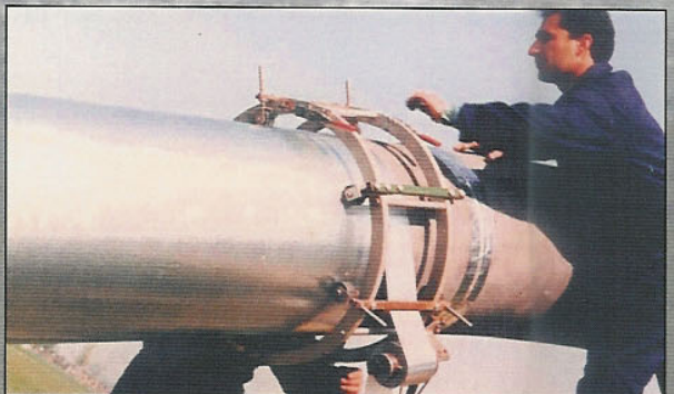
Application of zinc tape on above ground Pipeline.
