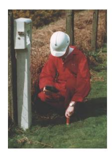
The test station consists of a preformed concrete post with a covered recess to contain a connection panel if required.
